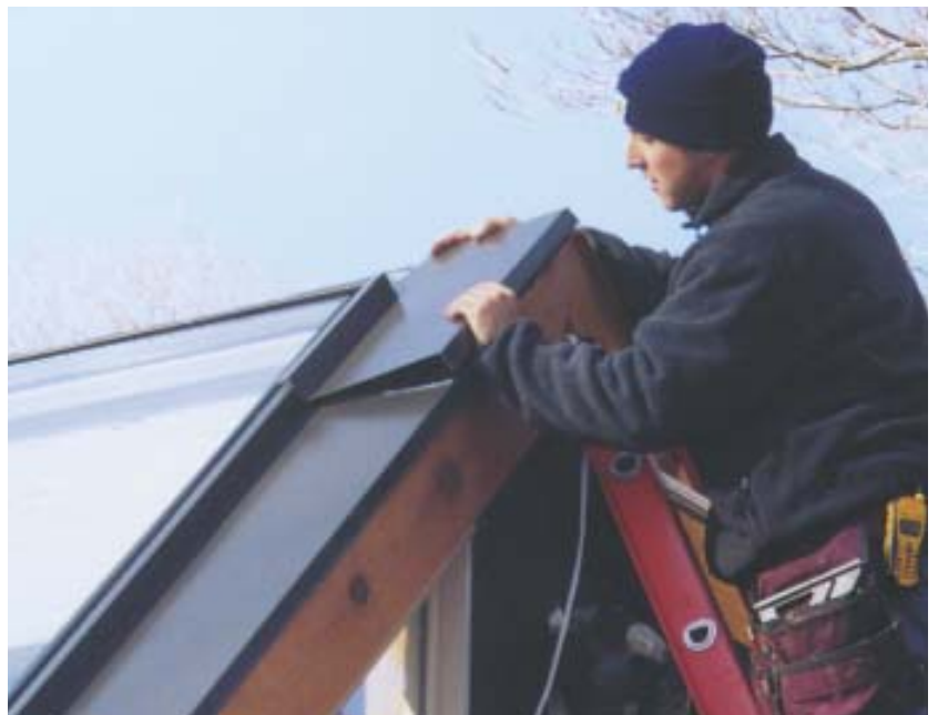
Figure 5. Because every overhead glazing job is different, flashings are custom-bent on site. The first installed is the eaves flashing (above), which goes on before any glazing bars. After the glazing is in place, the side flashings are installed (right).
