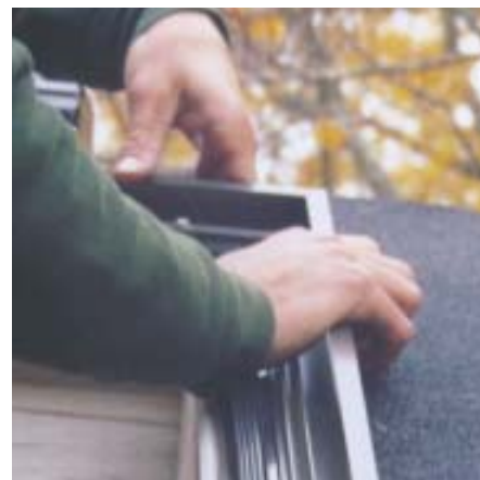
Figure 3. The crew used soapy water as a lubricant to help seat the gaskets in their raceways (left). Because the gasket material has memory, or a tendency to shrink back to its original form after stretching, it's important to install the gasket strips long and let them shrink for several hours before final trimming. The top perimeter bar is installed first, with mitered ends, then the side bars (below).
