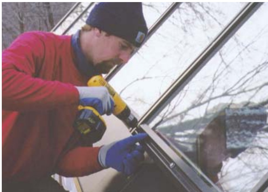
Figure 6. Attaching the gasketed glazing cap makes the installation watertight. A snap-on cover trim will hide the screw heads.
